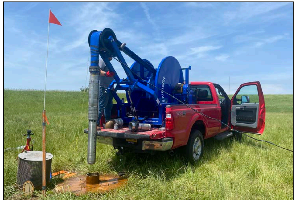
Multiple Well Pump Tests
