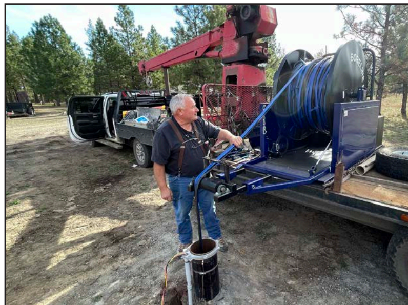
920 ft Pump Install
