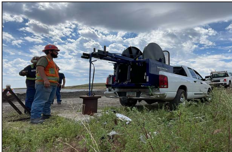
Speedy BOLT Mine Install
